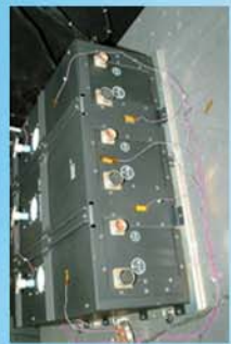
Six batteries Into Bays 2 and 3
