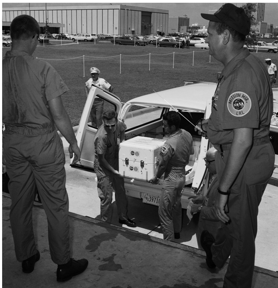
Figure 4.5 The first Apollo 11 sample return container is unloaded at LRL.
