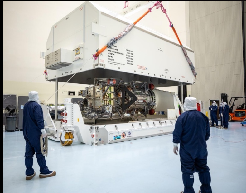
Shipping container opening in the Payload Hazardous Servicing Facility (PHSF) at KSC, following C-17 flight from March Air Reserve Base
